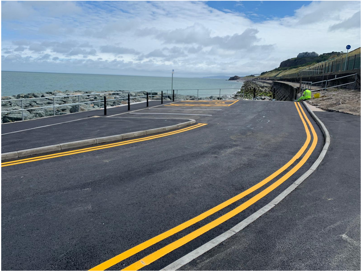
New surfacing and parking bays
